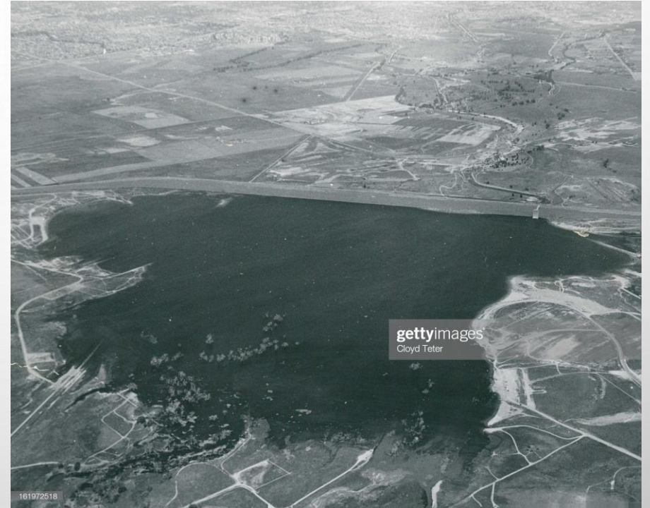
CHERRY CREEK RESERVOIR FOLLOWING DAM CONSTRUCTION
