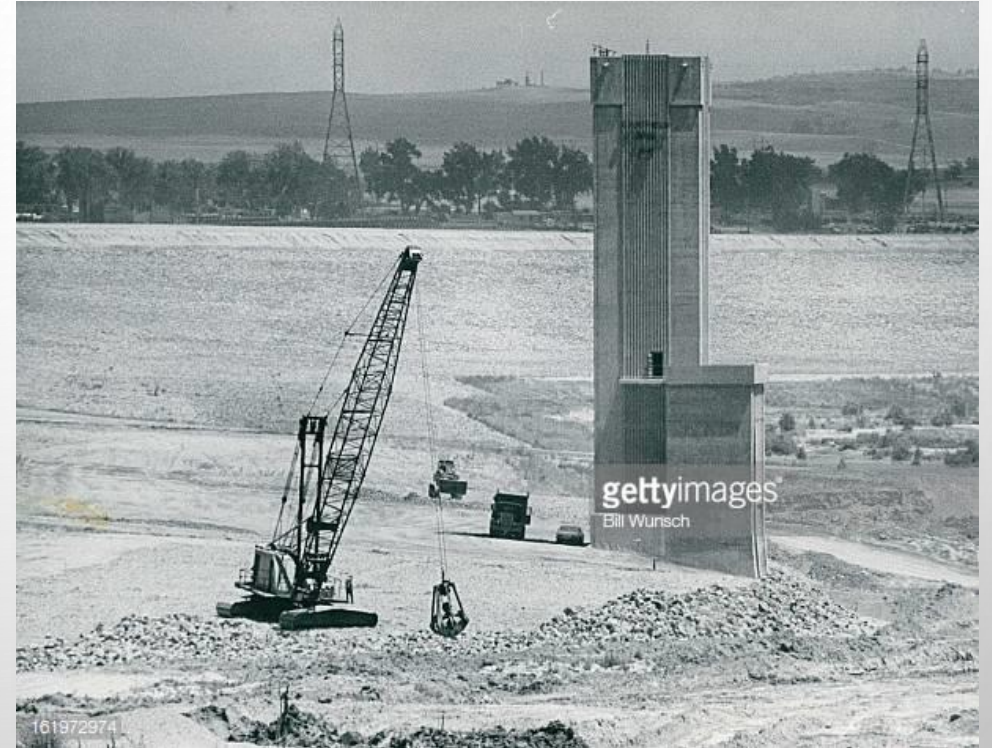
CHATFIELD DAM UNDER CONSTRUCTION
